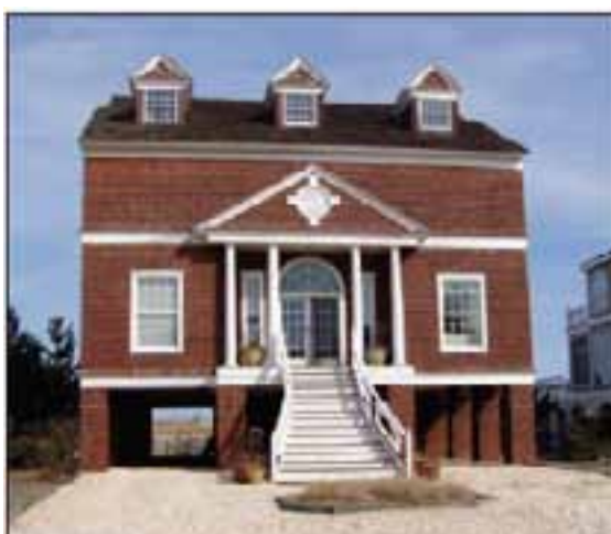
Coastal home elevated to avoid future flooding.
